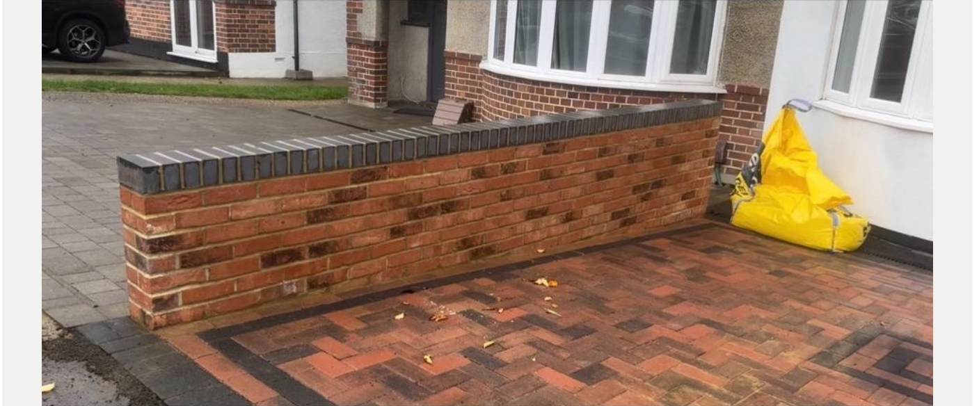
BOUNDARY WALL, DARK COPINGS AND PAVING EDGE
