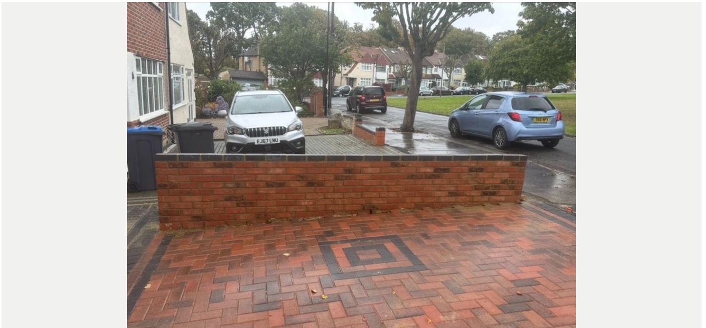
PAVING PATTERN AND CONTRASTING INSET DETAIL
