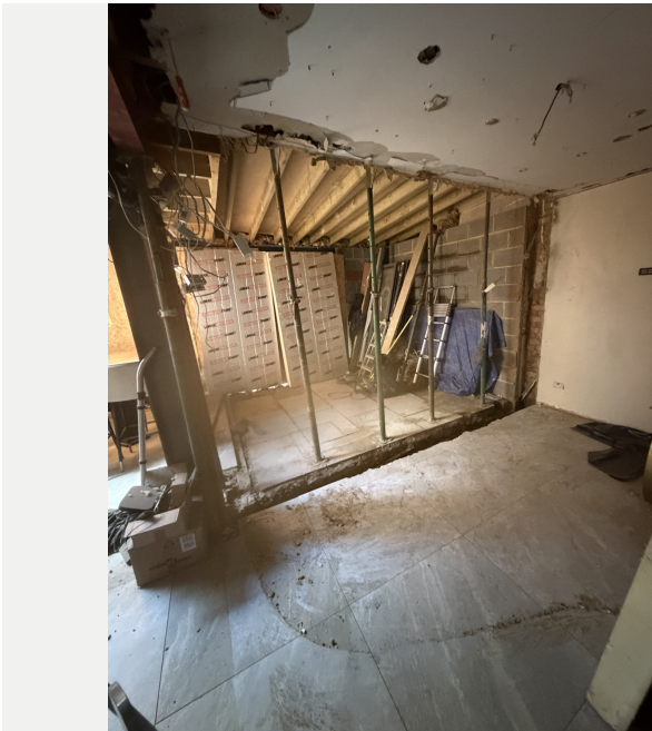
EXPOSED INTERIOR AND OPENING
