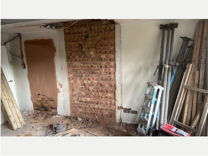
EXPOSED WALLS DURING WORK
